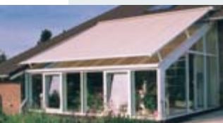
Vivienda conservatory with roof-mounted conservatory awning
